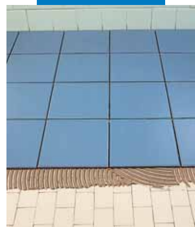
Tile on tile with Keraflex Grey
