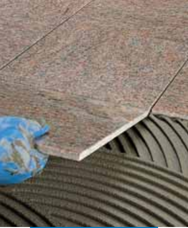
Installation of pre-glossed marble on floors
