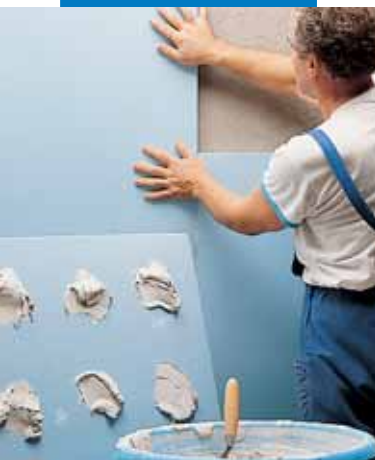
Laying polystyrene foam slabs with Keraflex white
