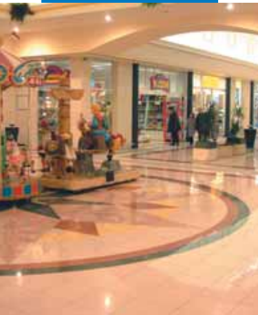
An example of an installation of porcelain tiles - Zanchetta Shopping Centre - Treviso (Italy)
